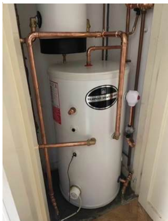
The upgraded indoor cylinder/ pipework
